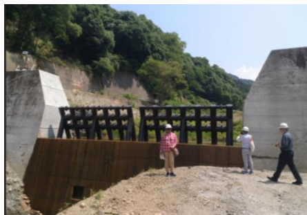
Closed dam was repaired to be an open dam for capturing more driftwood
