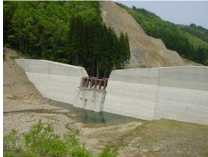
Partially-Open type sabo dam
