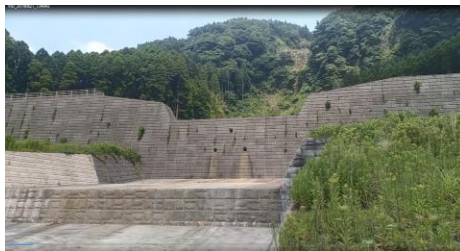
Closed dam, channel works behind the dam are needed, Kyushu, June 2019
