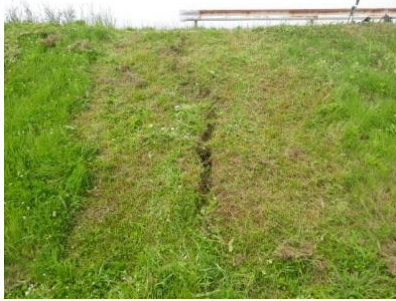
Slope gully corrosion repairs
